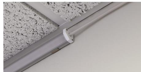
10. Use a ruler to place the mounting clips [included] near the location of the ends of the channels.
