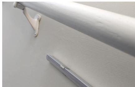
10. Secure the channel into the clips.
